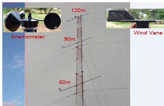
Figure 2 Wind mast and all equipments
