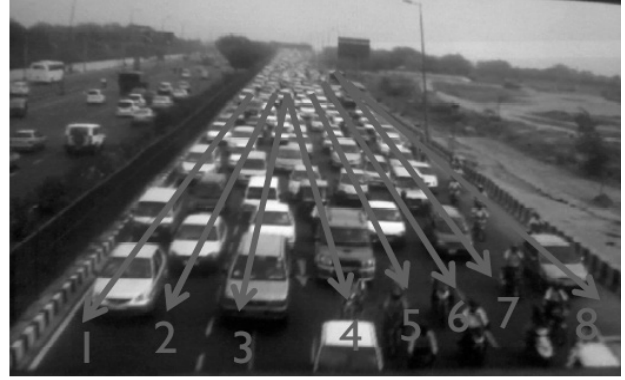
Figure 6 Vehicles travelling in eight virtual lanes on the divided urban expressway in India 11
