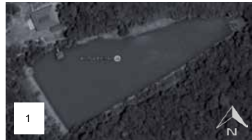
Figure 1 Huai Kasain reservoir Number 1 is structure of Floating PV.
