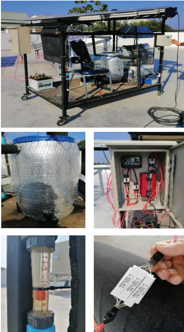
Figure 7 Examples of installed tools
