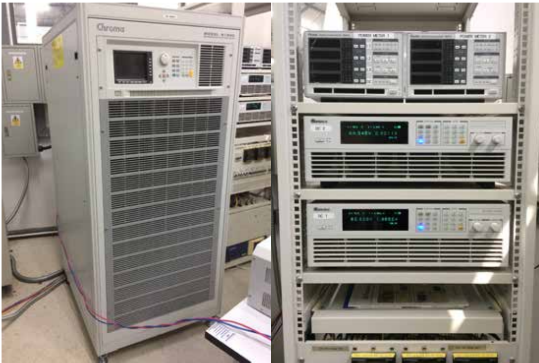
Figure 4 PV array simulator, grid simulator and digital power meter
