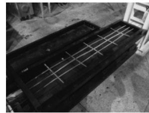
Figure 9 Finished Reinforcement in Form
