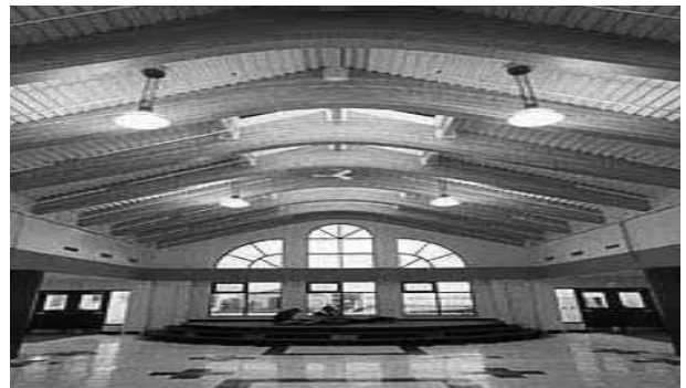
Figure 14 Curvature structure of glulam. 8
