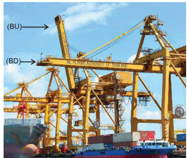
Figure 1 Working of ship-to-shore gantry crane (ที่มา: https://www.thadarat.com )
