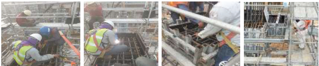
Figure 1 The setting anchor bolts use the electric welding cabinet. (before improving the work process.)
