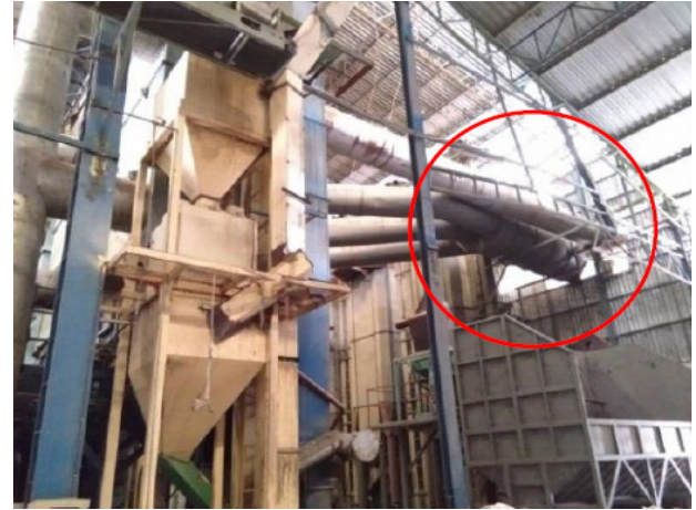
Figure 4 Installation of heat exchangers
