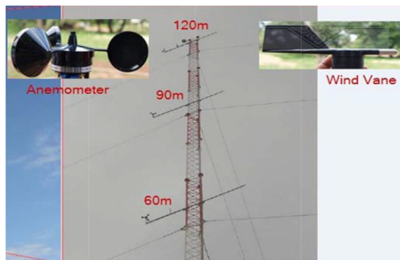
Figure 2 Wind mast and all equipments
